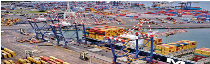
TPT will not be responsible for weighing containers when the new Solus regulation kicks in but will instead work on a pre-advise system.
